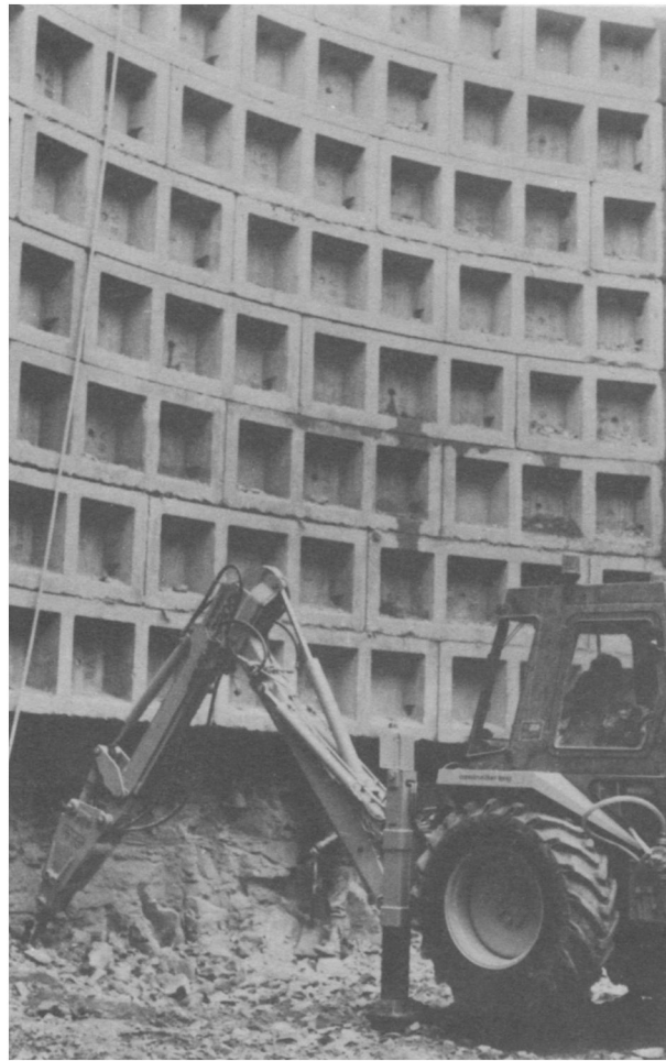
Fig 12. 19.0 m I.D. precast shaft rings at Seaton Valley, Tyne & Wear.
